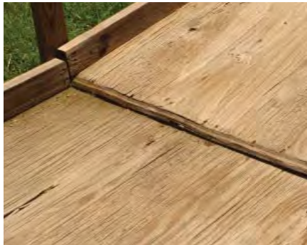
Uneven, bumpy transitions, warped slick surface.
