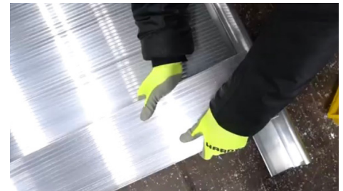
Quick and easy, 2 man team can build 60 feet ramp per hour
